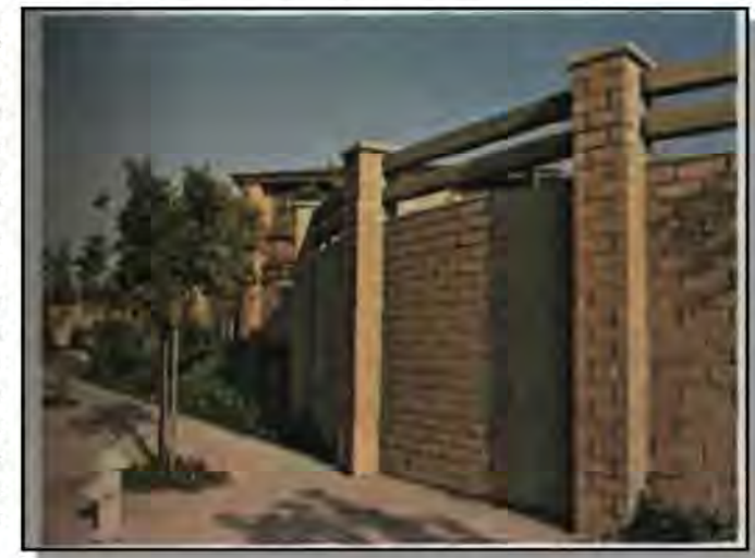
Figure 2 - Pilasters serve as vertical elements
